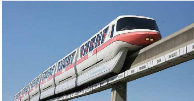
MONORAIL- OCTOBER Cable Trays
