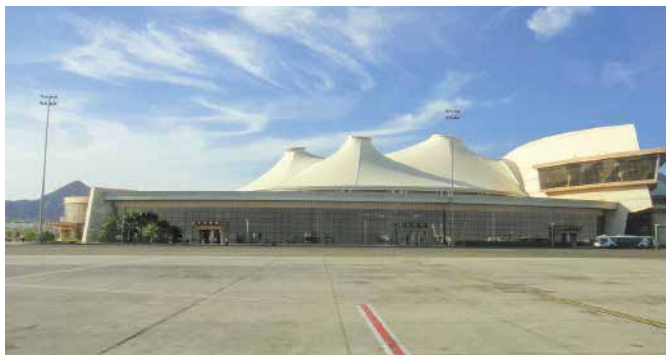
SHARM ELSHEIKH AIRPORT Power
