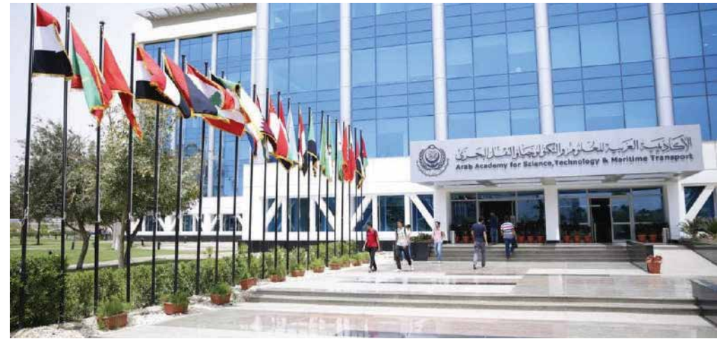
ARAB ACADEMY FOR SCIENCE AND TECHNOLOGY Indoor + Outdoor Lighting
