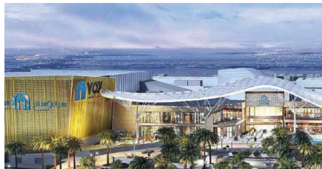
THE ALMAZA MALL ALFUTTAIM GROUP Cable Trays
