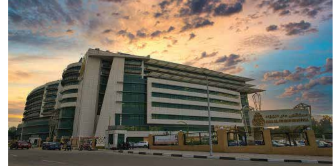
DAR EL FOUAD HOSPITAL Bus Trunking System
