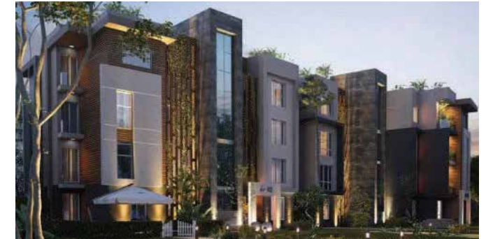
ACACIA COMPOUND Decorative Poles
