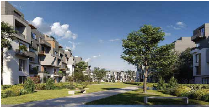
SODIC-EAST-NEW-CAIRO-COMPOUND Lighting Poles
